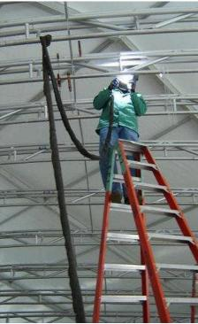
On the morning I was out at the site, the final trusses were being welded into place by some workers while others were working on the installation of some of the 24 exterior fabric panels.
